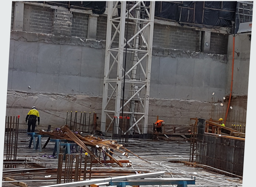
▲ 50mm Liteboard void form used with pier and slab
