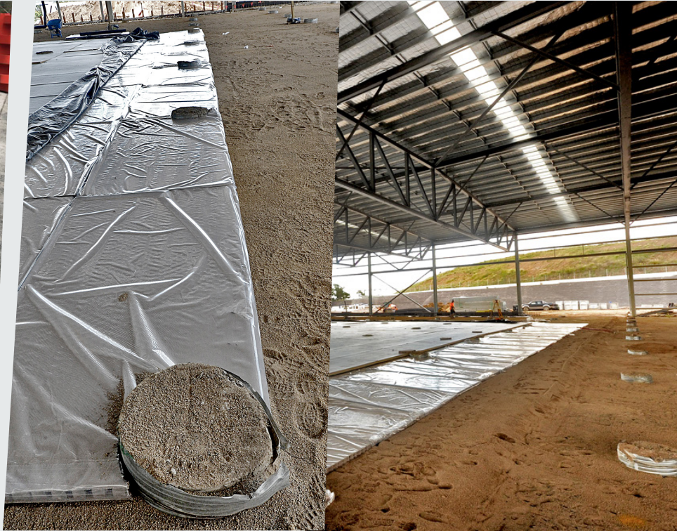
▲ 50mm Liteboard void form used with pier and slab
